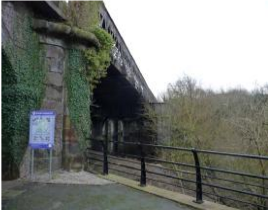
Dee railway bridge
